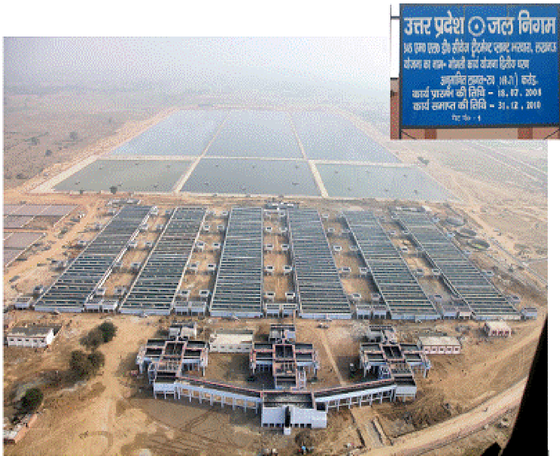
Aerial View of 345 MLD STP (UASB) at Bharwara
